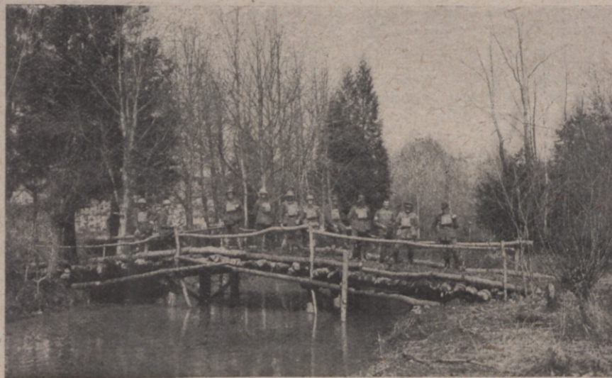
Bridge Built by Australian Engineers.
