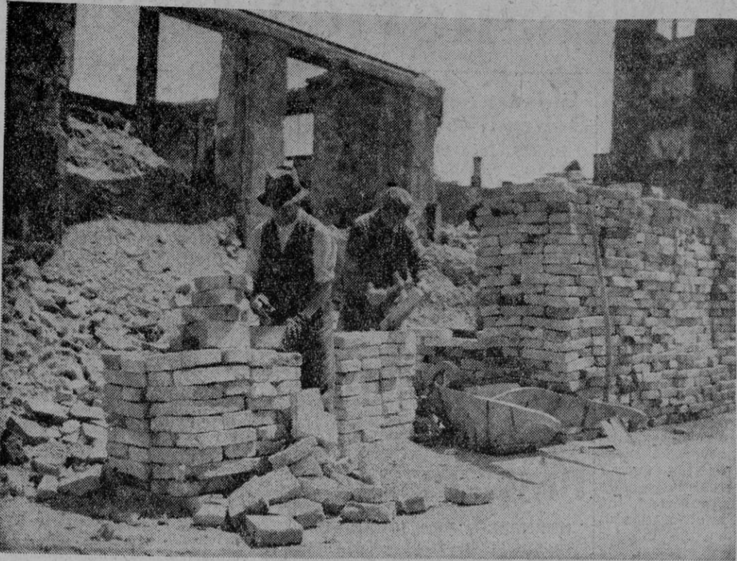
MUNICH contractors salvage bricks to be used in the reconstruction of bombed areas. Other German cities are in a similar stage of initial rebuilding. Materials used are German, with contractors being licensed by the economic division, military government.
