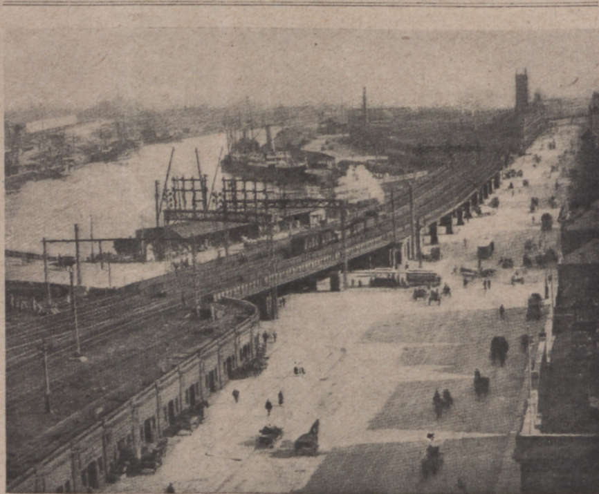
The recently finished duplicated railway viaduct which connects Flinders and Spencer Street Stations, Melbourne.
