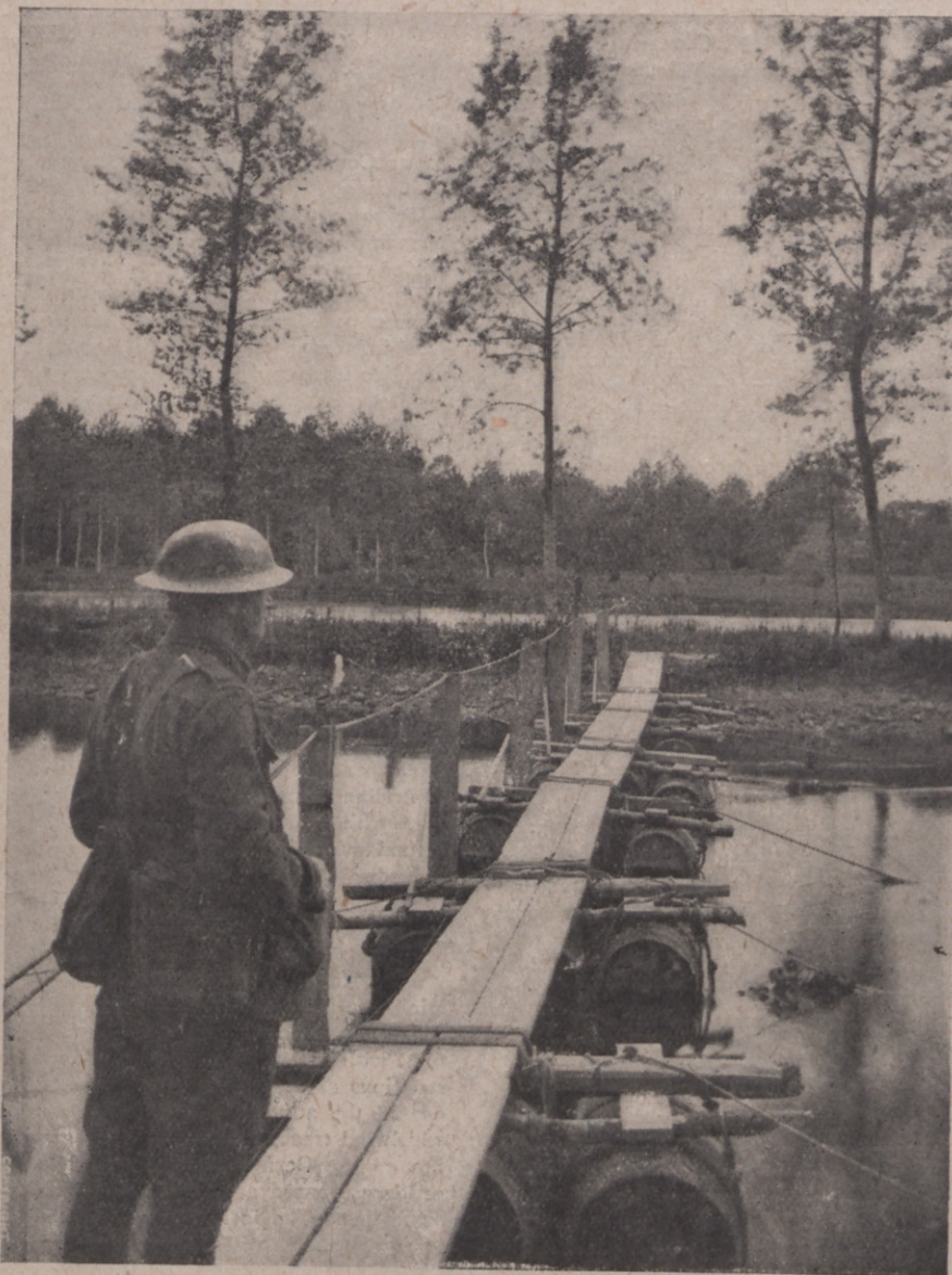
A Two-Plank Barrel Bridge Built by Australians.
