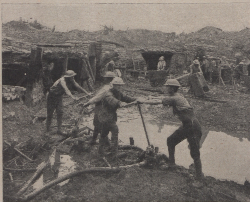
The Australian Tunnellers making Dug-outs. Most of these men are miners and are doing magnificent work. They are here seen pumping out the soakage.
