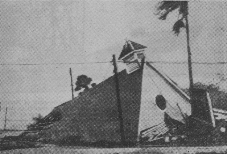
The storm battered this Port Lavaca church, knocking it askew and ripping off and scattering the clapboards. Note cross set awry.
