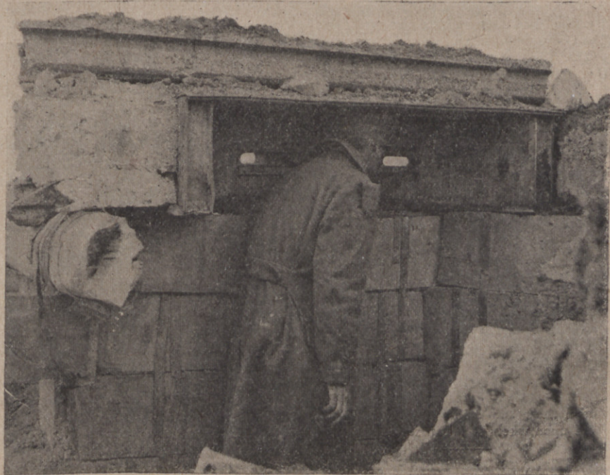
A machine-gun emplacement, though solidly built with slabs of concrete, supported by heavy timbers, was effectively strafed by our heavy guns. (Australian Official Photograph.)
