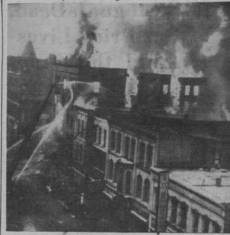
In Lima, Ohio, firemen pour water into the Milner Hotel (formerly the Norval) as the structure went up in flames, two weeks ago. Three other buildings also burned in same fire.
