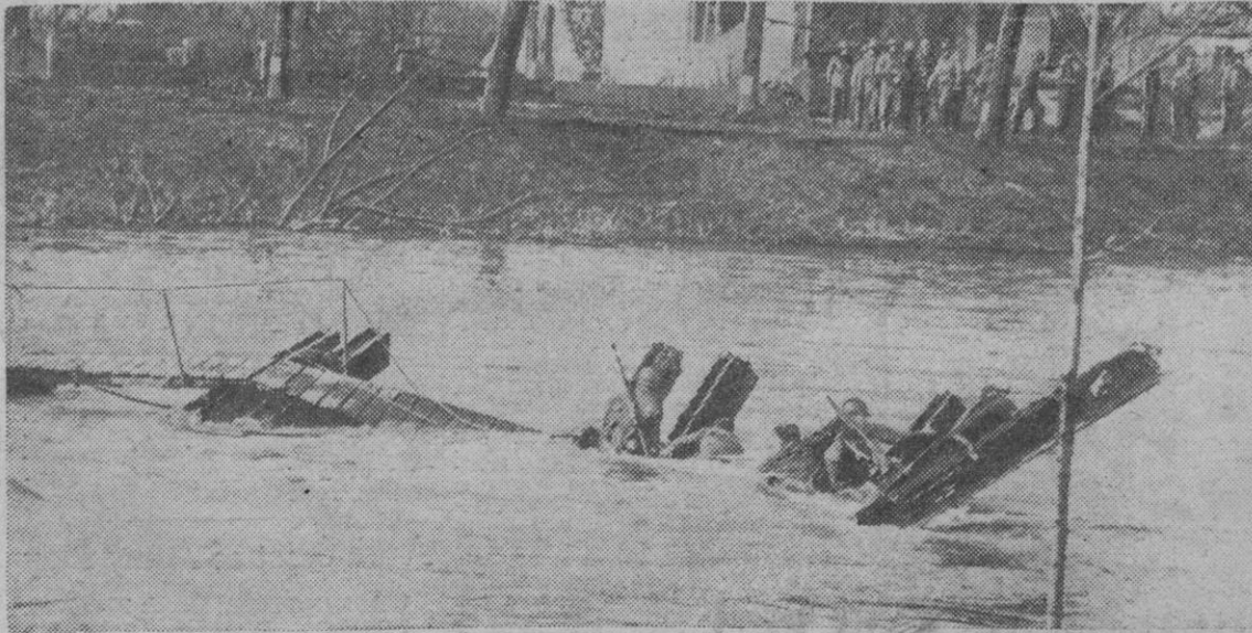
A temporary footbridge over the Roer River collapses under the weight of two stretcher-bearers carrying a wounded Yank and the body of a soldier killed during crossing operations. Other Yanks on the shore tensely watch as the soldiers struggle in the swirling waters.
