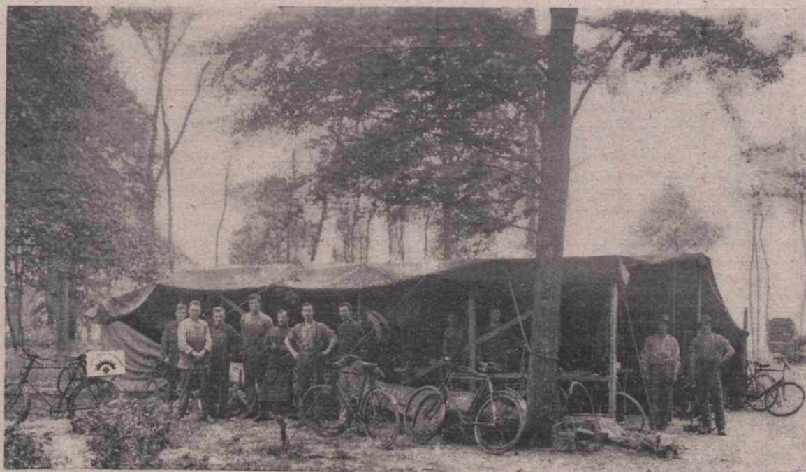
Repair shop of an Ordnance Depot in France.
