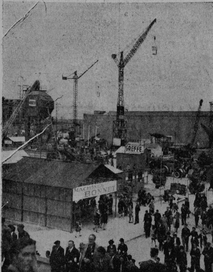
CONSTRUCTION equipment displays drew large crowds. Exhibits were set up by manufactures from many countries.
