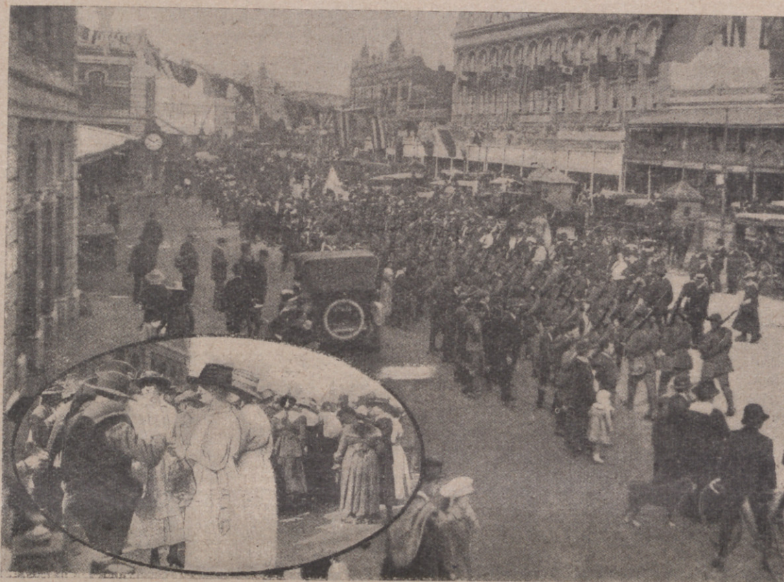
A.I.F. Troops at Perth Central Railway Station. Crowds cheered these big, sturdy men from the West.
