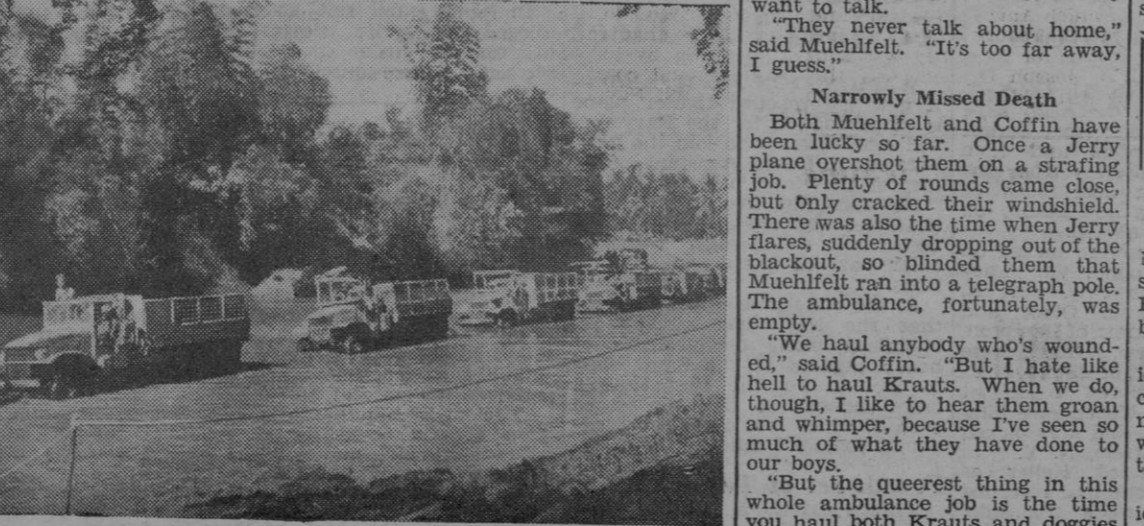
When Japs blew bridges on Luzon these six-by-sixes took to the tropical waters of a river near Lingayen. The Nipponese did a very thorough job of destroying their bridges behind them but this failed to stop the U.S. columns from pouring into Manila from several expanding beachheads by wading across water barriers.
