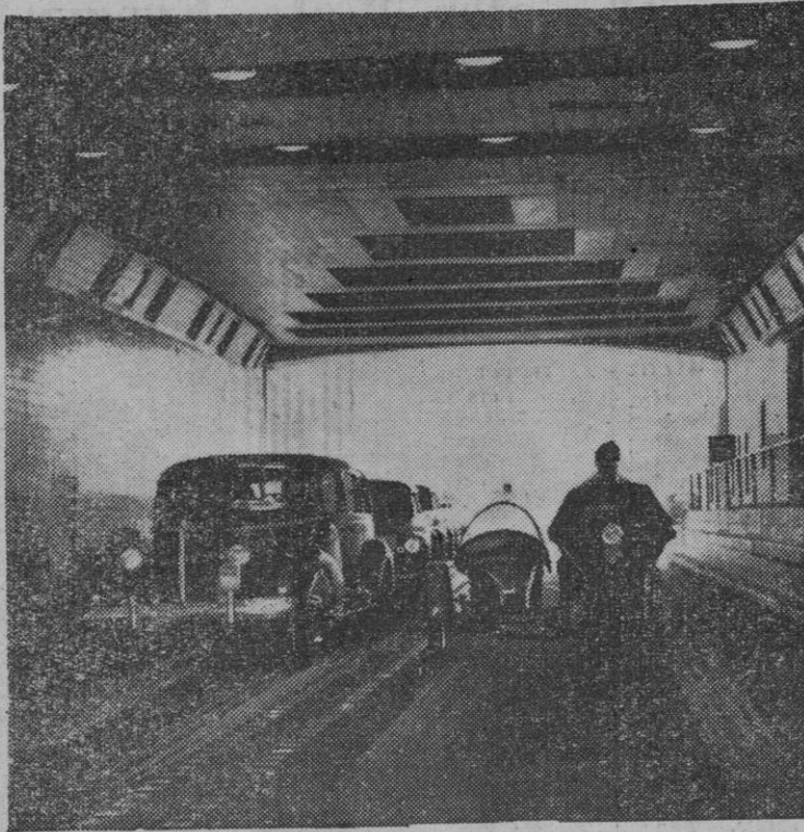
With the opening of the new tube of the Lincoln Tunnel between New York and Weehawken, N. J., two one-way passages are provided under the North River. Official cars are shown entering the new section, which opens between W. 39th and W. 40th Streets on the New York side. The first tube was completed in 1937.
