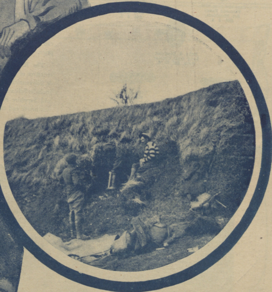
Australians Digging a Gun Emplacement.
