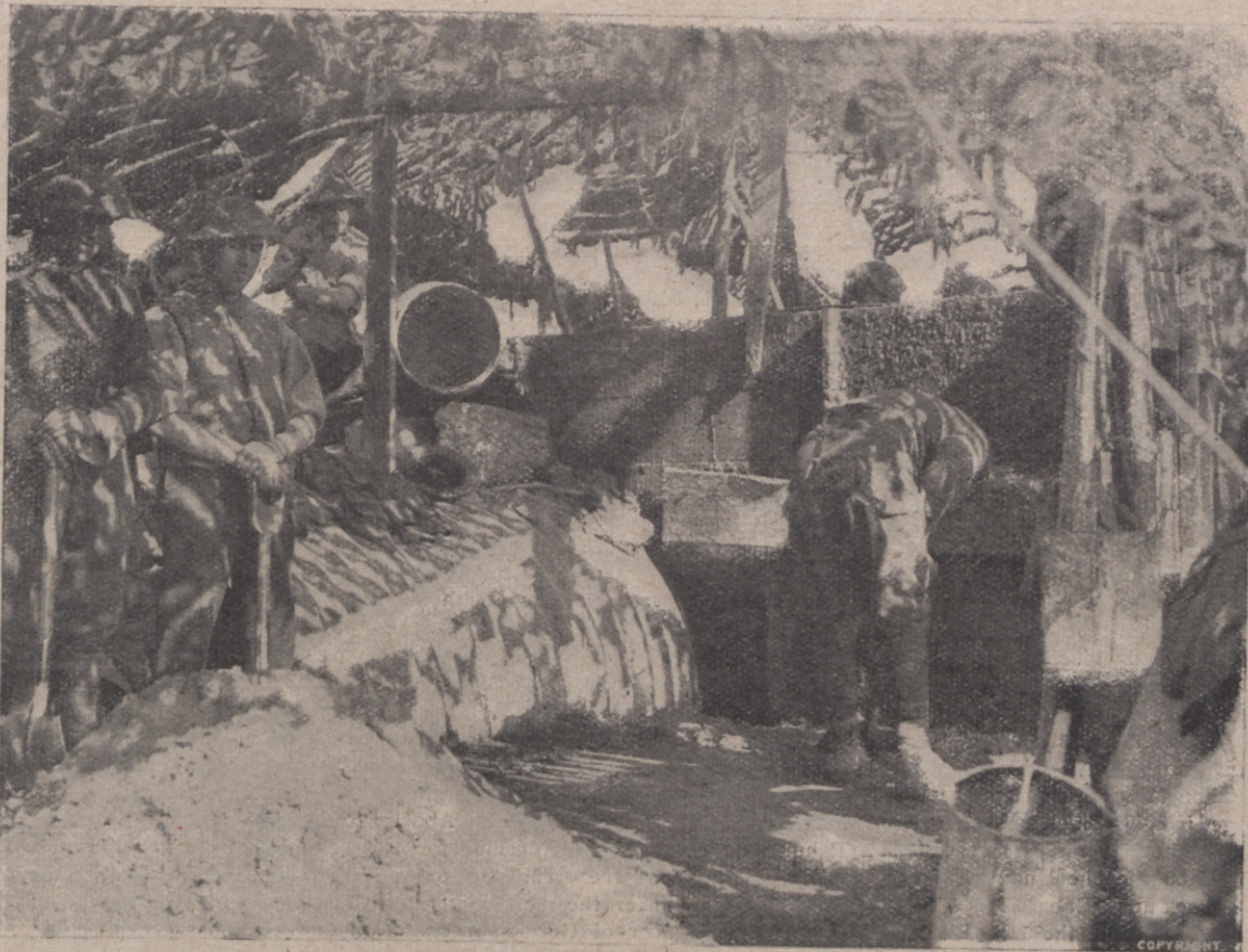
Making a reinforced concrete shelter under camouflage.
