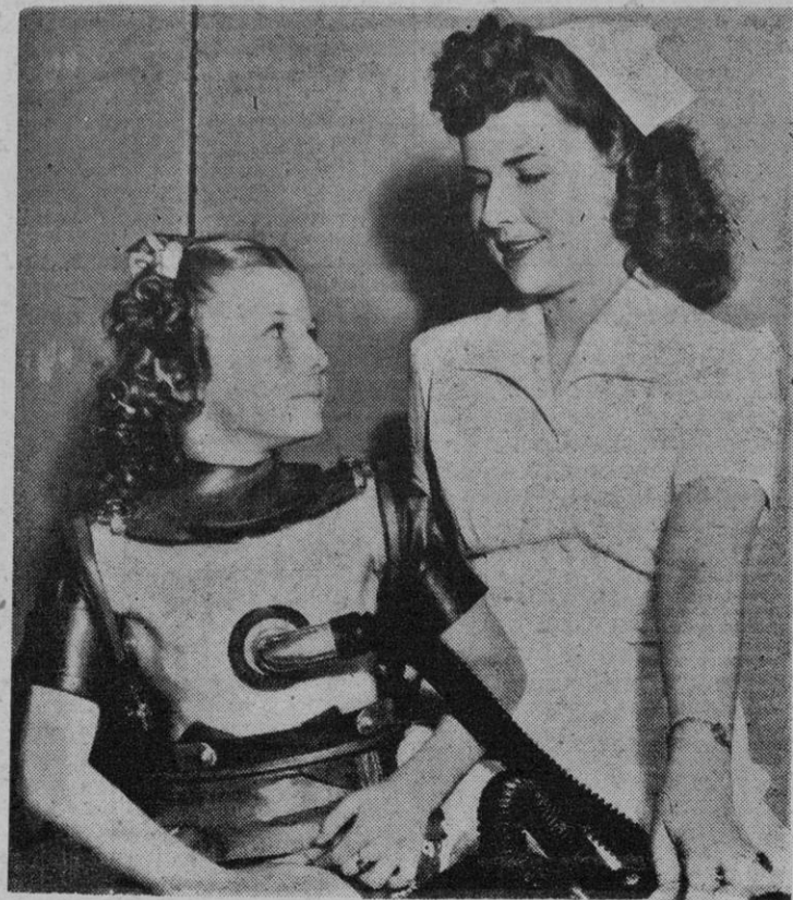
NURSE MINNIE MALEK adjusts a new portable plastic "lung" weighing less than 60 pounds on patient Barbara Johansen. The new device will be a boon to infantile paralysis victims who are now using the heavy iron lung weighing from 600 to 2,300 pounds.
