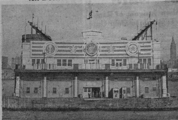
Six piers at the New York POE got a face lifting as part of the program for welcoming returning veterans. This offshore view shows the North River end of Pier 84, with the Empire State Building in the background.
