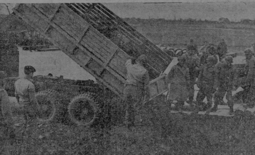
Aviation engineers fill bomb crater before laying the surfacing of new runway at one forest Allied airstrips in Germany. A few days after photograph was made Ninth Air Force fighter-bombers were using strip.
