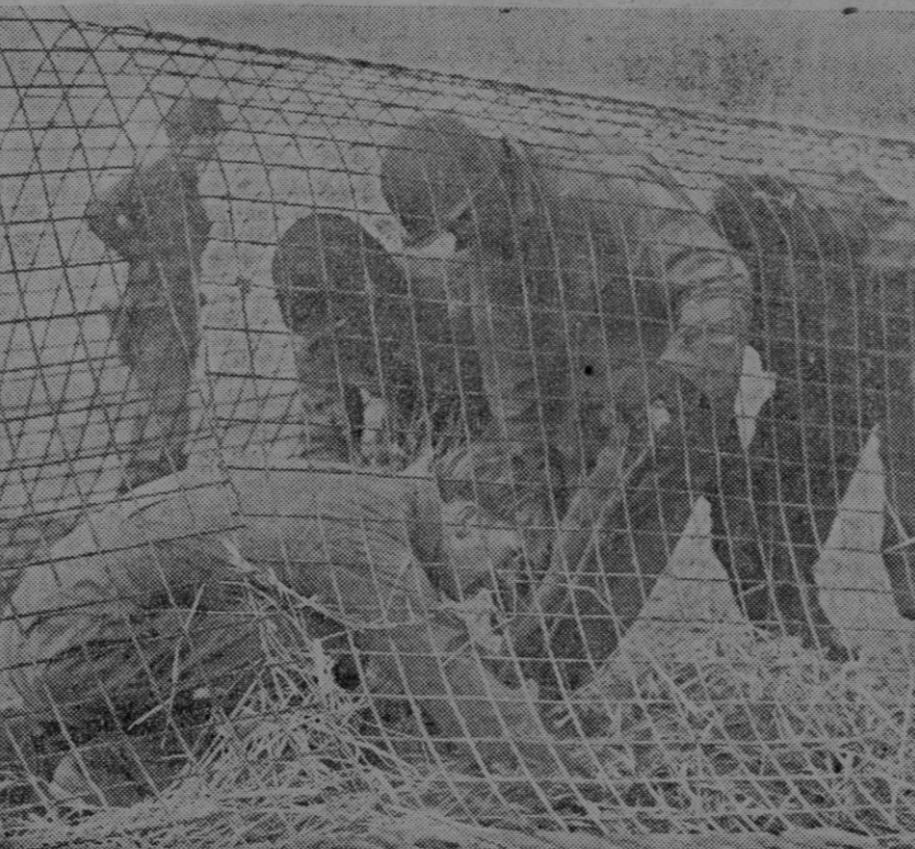
Soldier-engineer spreading straw under wire mesh. Straw will keep mud from forcing way through mesh when thaws set in.
