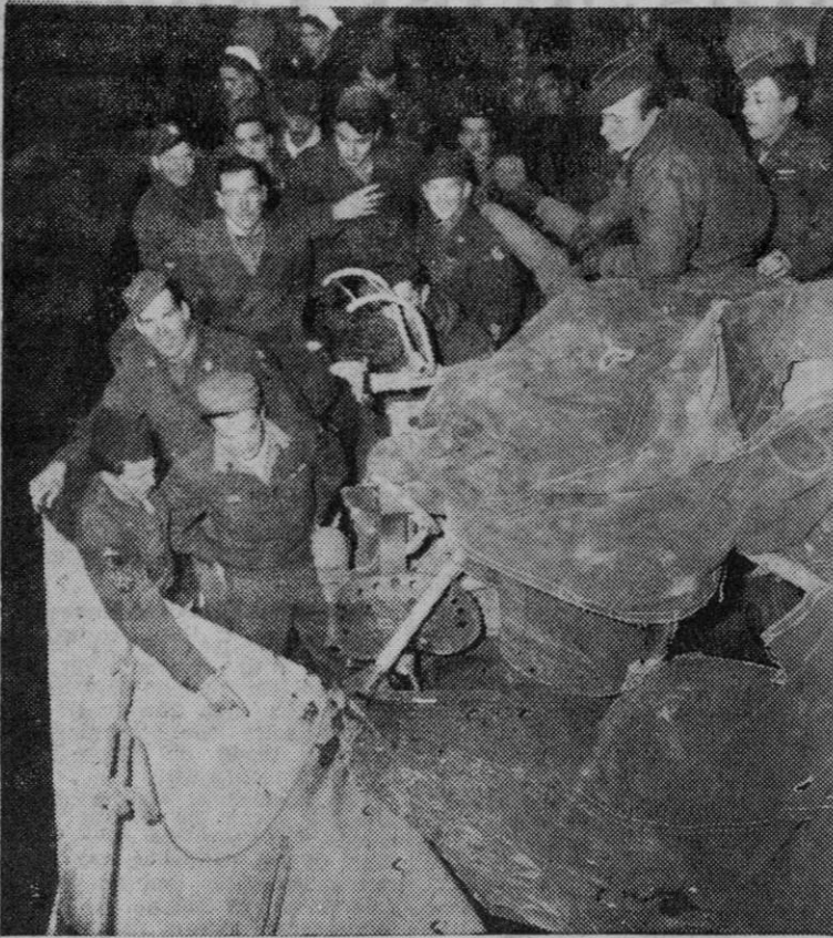
GIs survey storm damage to the cruiser Portland after it docked and discharged 1,000 soldiers in New York. Two GIs were killed and 22 were injured by the storm on the Atlantic crossing.
