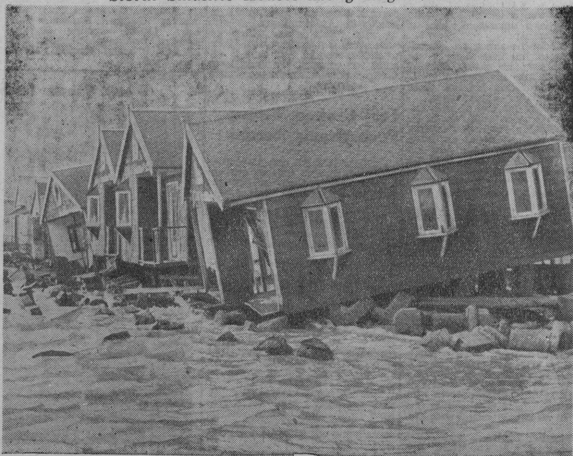
These bungalows in the village of Jaywick, east of Clacton-on-Sea, in England, were smashed in a recent tempest which swept across the British Isles. Heavy damage to other coastal towns resulted.
