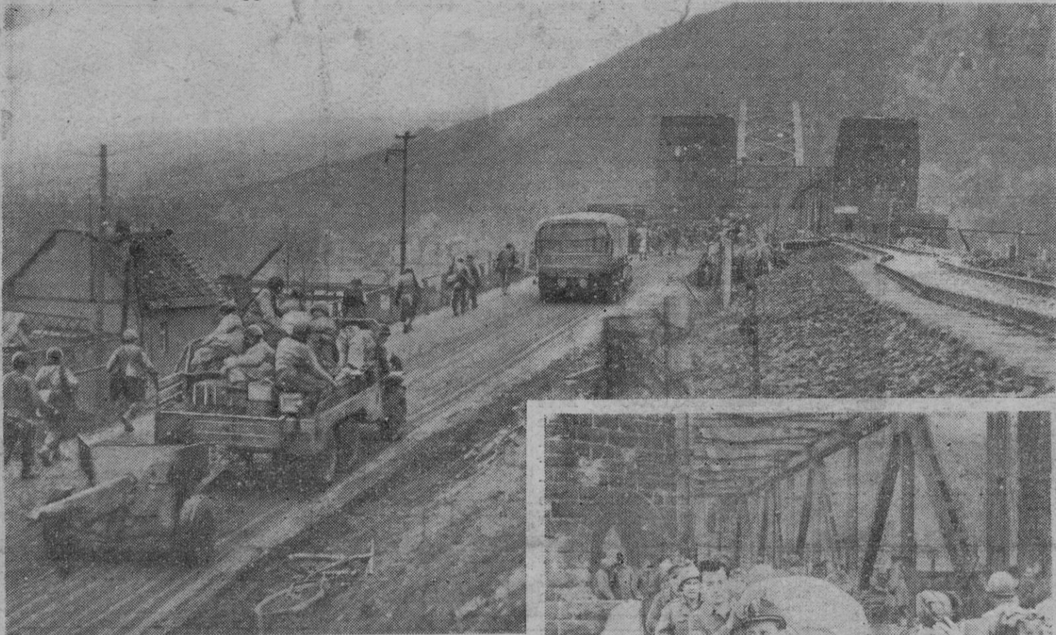
Supplies, men and equipment pour over the Ludendorff Bridge—the steel link across the Rhine won four days ago by the Ninth Armored Div. Erpel, a German village on the east bank, lies to the left. (Other pictures of the Rhine crossing on Pages 4 and 5.)
