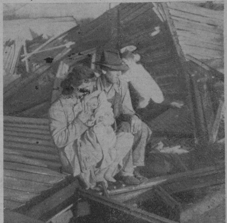
In Montgomery, Ala., Mr. and Mrs. O. M. Levinshold and their three-month-old daughter sit atop their demolished home after a twister had struck the area. All three crawled out of the ruins without a scratch. The storm occurred Feb. 13.
