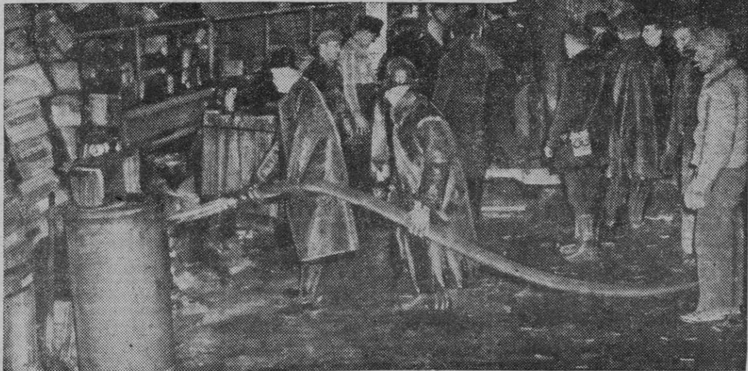
TRAFFIC JAM: Traffic in the Holland Tunnel, N. Y., was tied up for three hours as firemen battled a blaze caused when a truck caught on fire in the tube. The truck was carrying a load of chewing gum, and the job of clearing away the melted gum was more of a problem than the fire.
