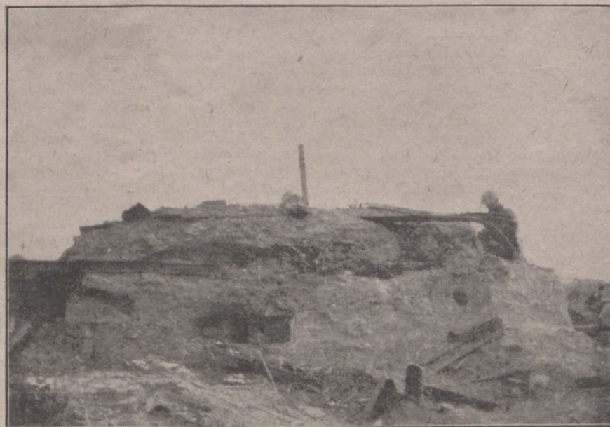
An old German "Pill Box" shelter, showing machine-gun emplacement. Note the steel in its concrete construction.
