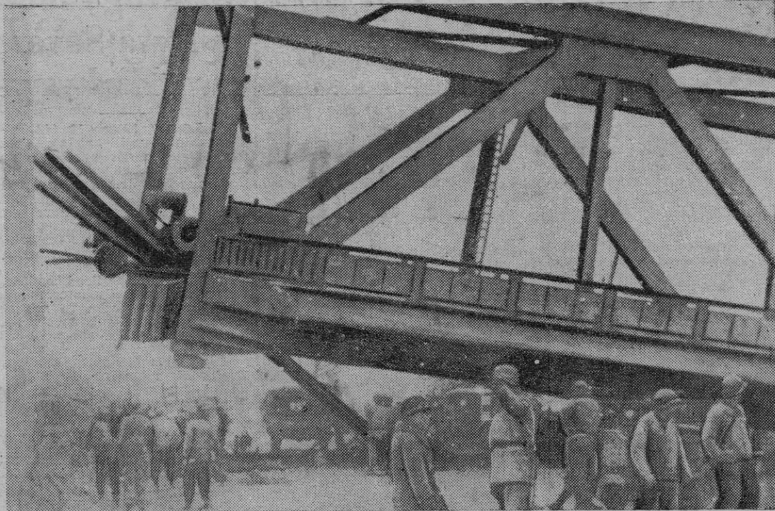
Closeup of one section of the fallen span.
