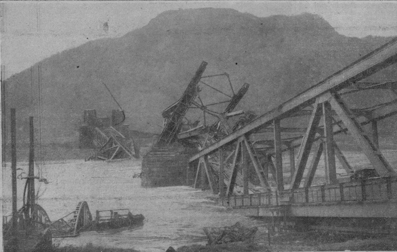
This is how the Ludendorff Bridge at Remagen, Germany, looked when an Army Signal Corps photographer reached the site shortly after the bridge collapsed last Saturday. The span was weakened by constant shelling and heavy traffic.—(Other Pictures on Page 3.)
