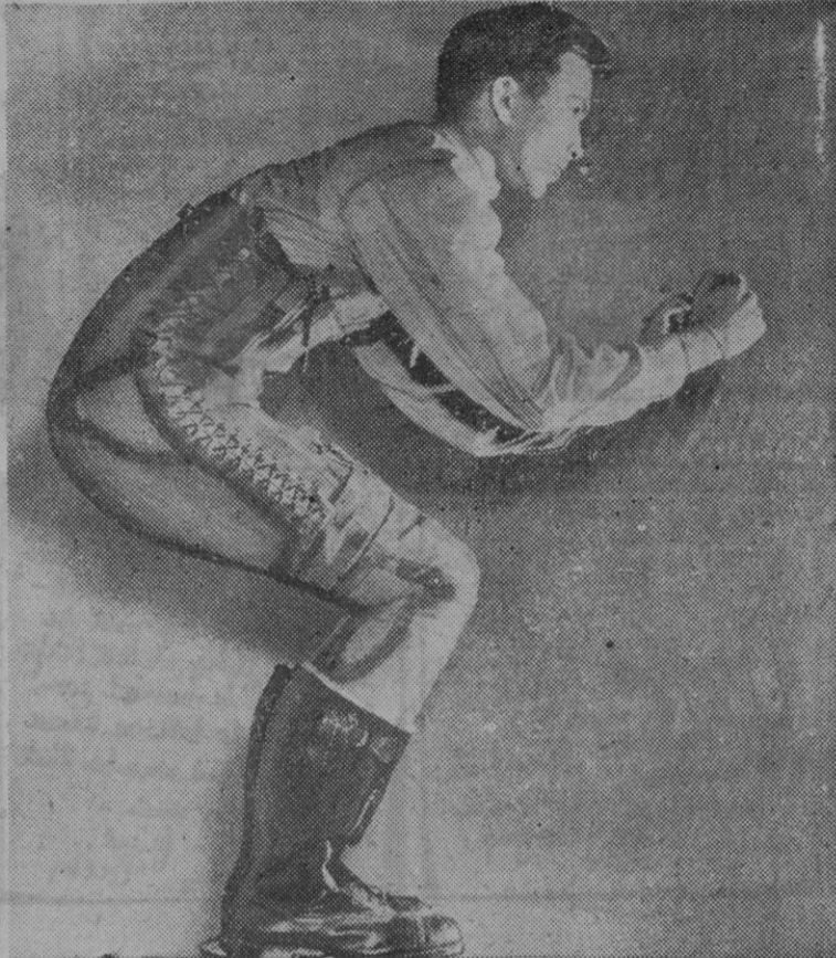
A Canadian airman shows how the new anti-blackout suit is to be worn by fighter pilots. Note how accurately it conforms to body contours in the sitting position. In use, columns of gas or fluid contained in the rubber lining exert compensating pressure permitting normal blood circulation to the brain.
