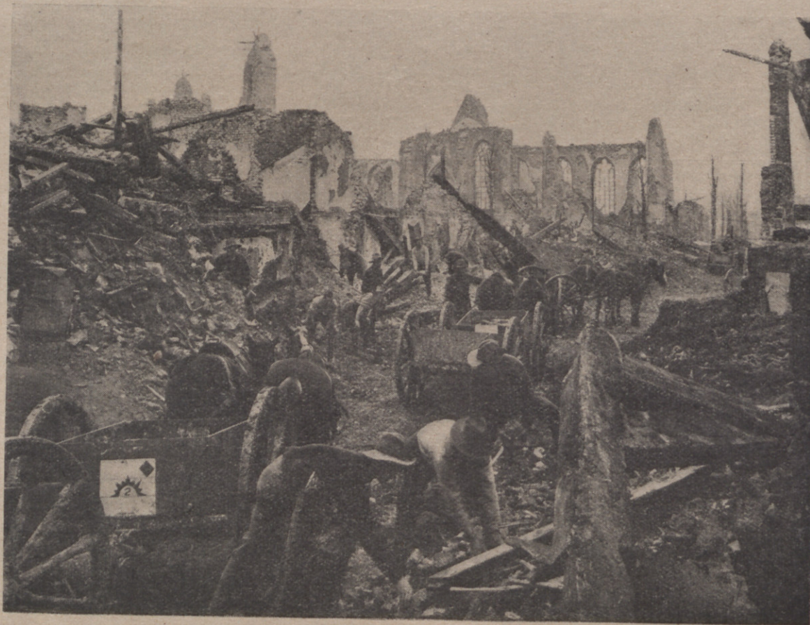
A railway gang taking bricks and stones for road and railway ballast purposes.
